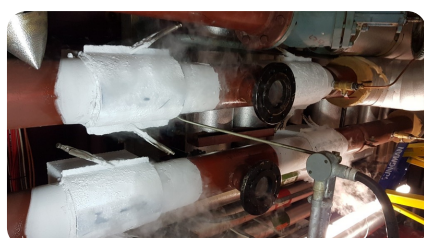
Pipe Freezing no line shutdown
